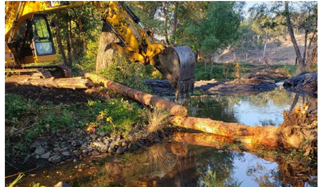
Large wood placement at Salt Creek river mile 3.5.
