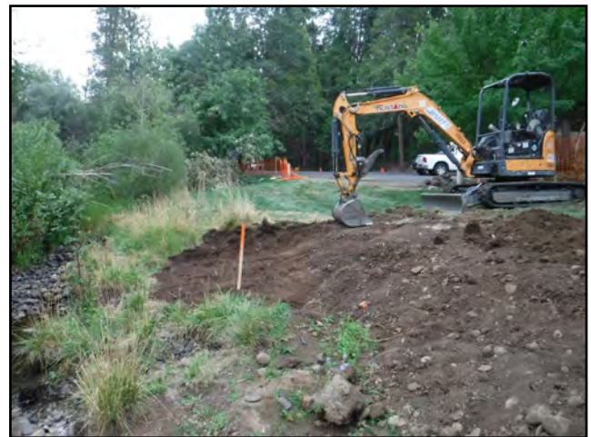
Reshaping the slope to a gentler grade
