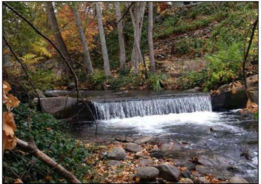
Upper portions of Ashland Creek provide excellent cool-water rearing habitat for juvenile steelhead, but fish movement from Bear Creek and lower Ashland Creek into these better conditions is blocked by the Smith-Myer-Roper Dam. With removal of this dam, visitors to Lithia Park could be greeted by the presence of much greater numbers of adult and juvenile steelhead and perhaps, Coho Salmon.
