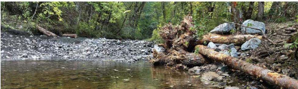
Harboldt Dam site after removal and placement of large wood structures.
