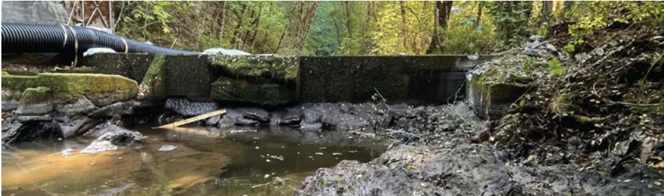
Harboldt Dam site prior to removal.
