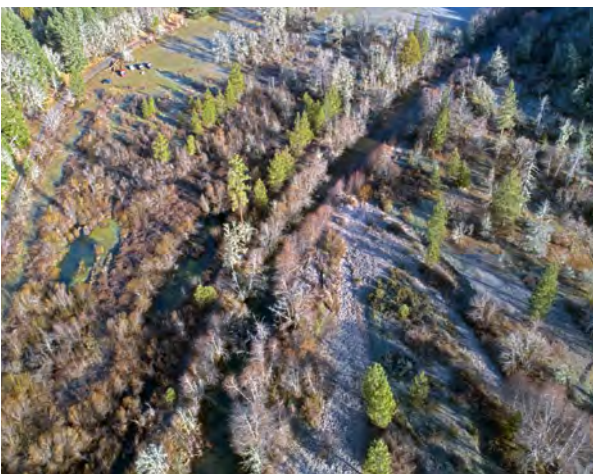
Bird's eye view of our largest project in 2020 at Elk Creek river mile 5.6 where large wood placements and strategic excavation allows side channels and the floodplain to reconnect with the stream channel.
