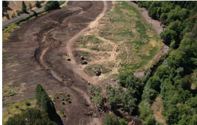
Construction during seasonal side channel reconnection.
