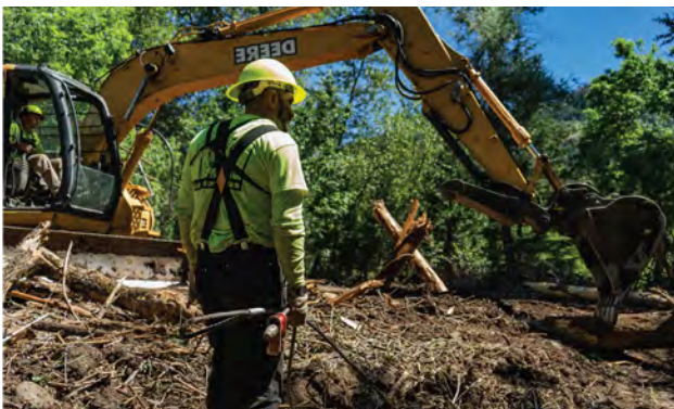
M&M Services installing large wood in the side channel.
