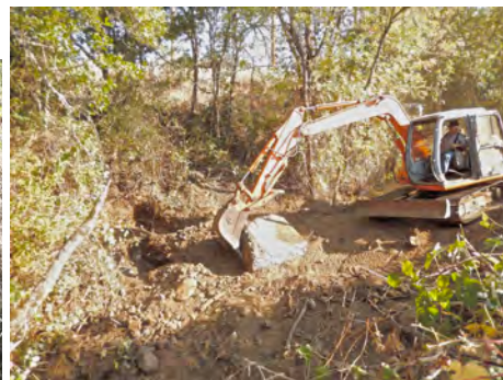
Concrete dam being removed (August 2015).
