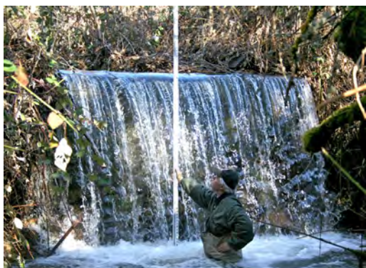
The dam on East Fork Jones Creek created a 9' jump for upstream migrating fish.
