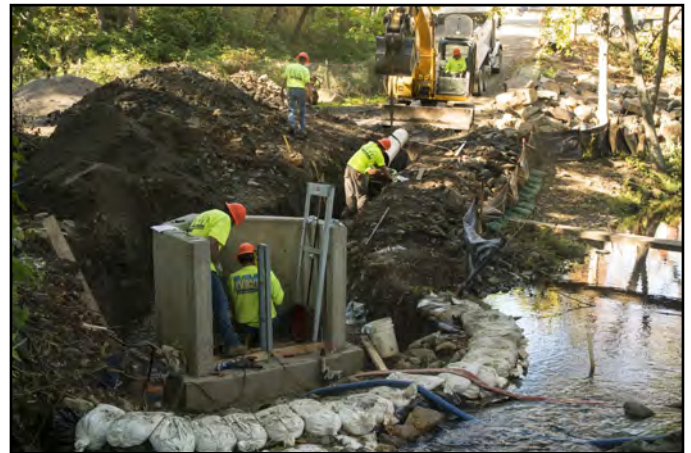
Newly constructed irrigation intake box
