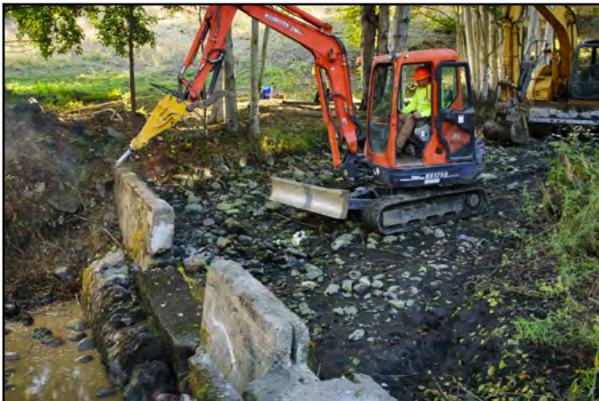
M&M Services, LLC begins demolition of the dam
