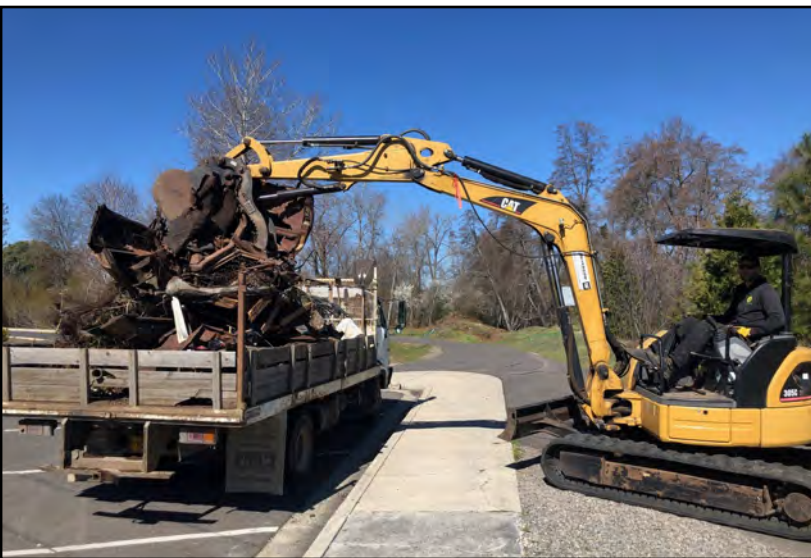
Some of the debris hidden under blackberries along Bear Creek
