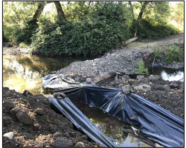
Photo: Both the push-up dam and concrete sill seen here will be removed and replaced with a new irrigation system that allows for juvenile fish passage during spring and summer.
