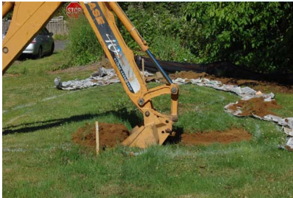
Figure 18: Excavator is located outside of the rain garden to remove soil to make sure the machine does not compact soil in the rain garden.
