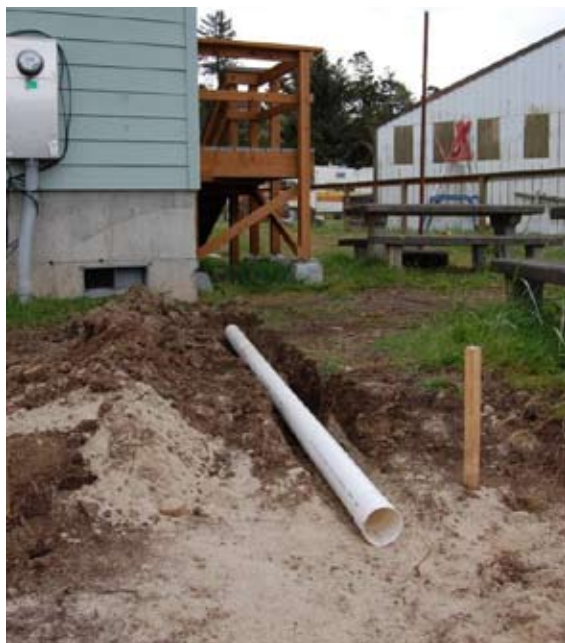
Figure 22: Four-inch ABS pipes here will convey water from this building into a rain garden. Pipes like these must be graded to drop about 1 inch for every 10 feet so that water flows away from the building but does not build up too much velocity by the time it arrives in the rain garden. (Photo: Robert Emanuel, OSU)
